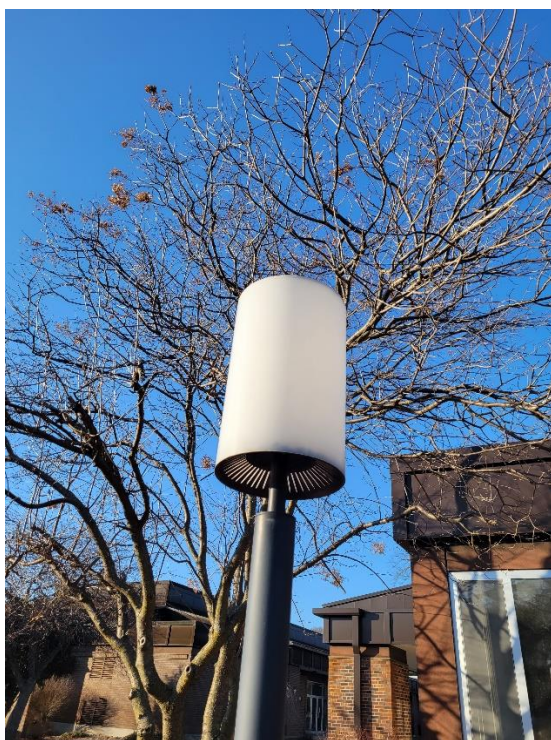
FIGURE 2 WALKWAY LIGHTING AT CAMPUS SITE (NOTE COMPLETE LACK OF SHIELDING)
