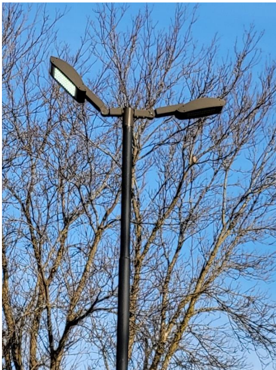
FIGURE 1 - PARKING LOT LIGHT AT CAMPUS SITE(NOTE ANGLED ORIENTATION)
