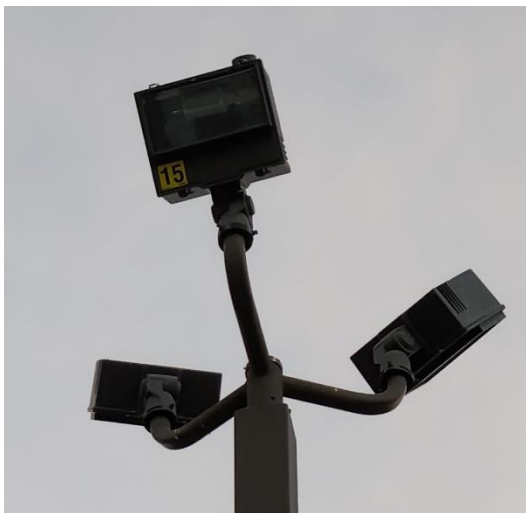
FIGURE 12 TYPICAL POLE MOUNTED ANGLED FLOOD AT THE HIGHWAY SHOP SITE
